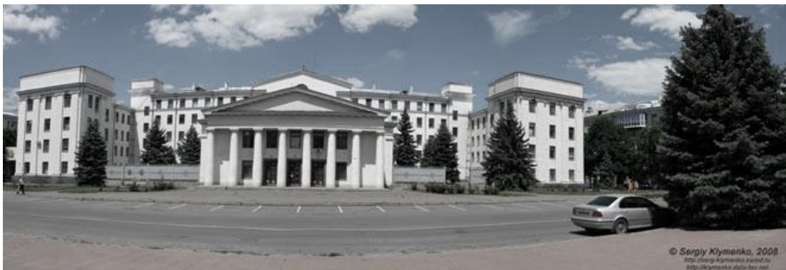
Building of the Regional State Administration in Luhansk [151]
