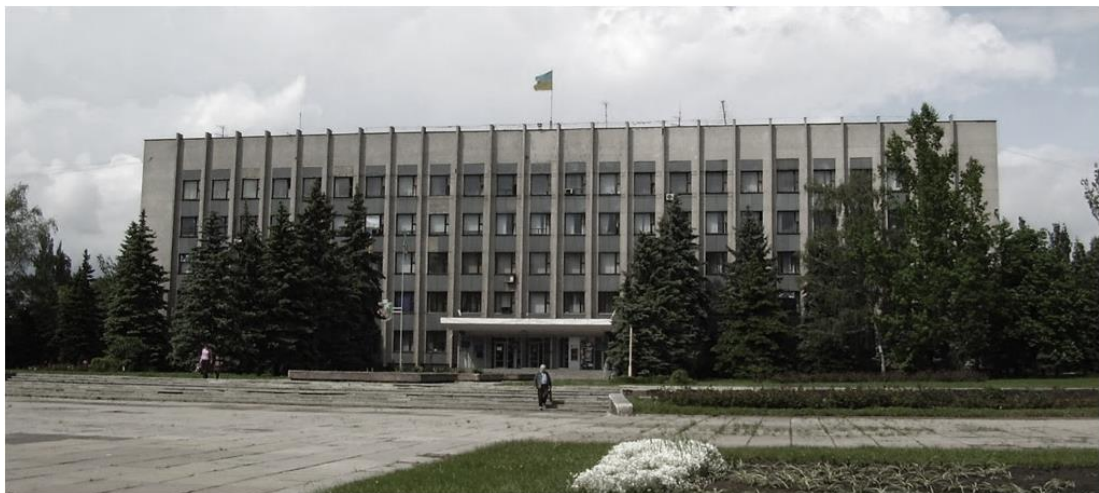
Administration Building in Horlivka [136]
